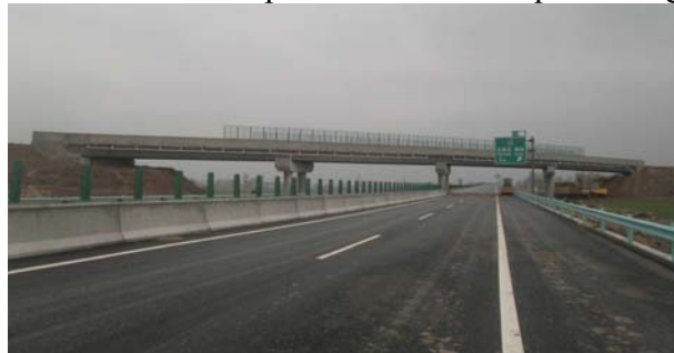
Figure 4 The First Completed UHPC Highway Bridge in China
