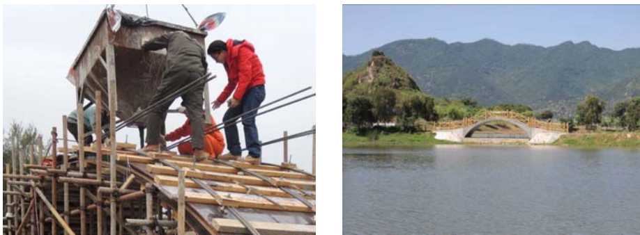
(a) Under construction
