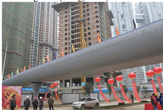
Figure 7 The UHPC Pedestrian Bridge in Changsha
