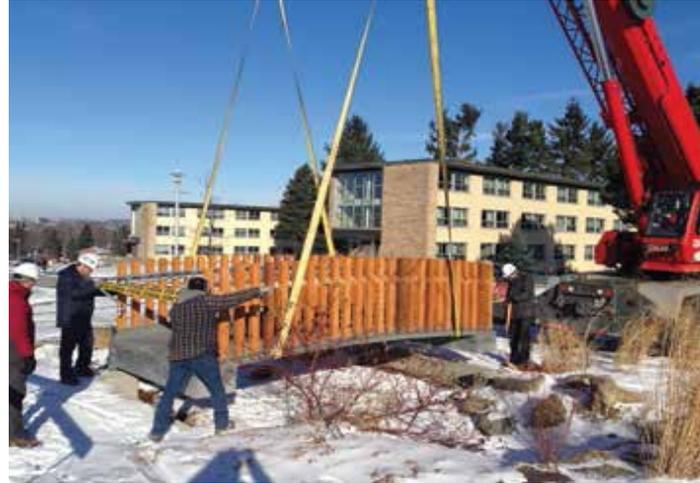
Figure 2. UHPC Footbridge Built at the University of Sherbrooke
