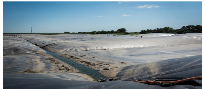
Figure 1. Impermeable cover on a manure storage that allows collection of biogas, keep rainwater out of the manure, and help minimize odor and ammonia loss, but is it ever cost feasible?
