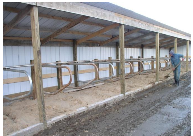
A single row of 33 cow-tels with 4'x9' stalls built for less than $300 per stall without labor. Cow-tels are open to the south but somewhat protected by a building 14' to the south. Stalls are sand bedded.
