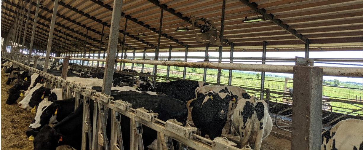
Figure 2. A combination of recirculation fans and sprinklers to provide cow cooling.
