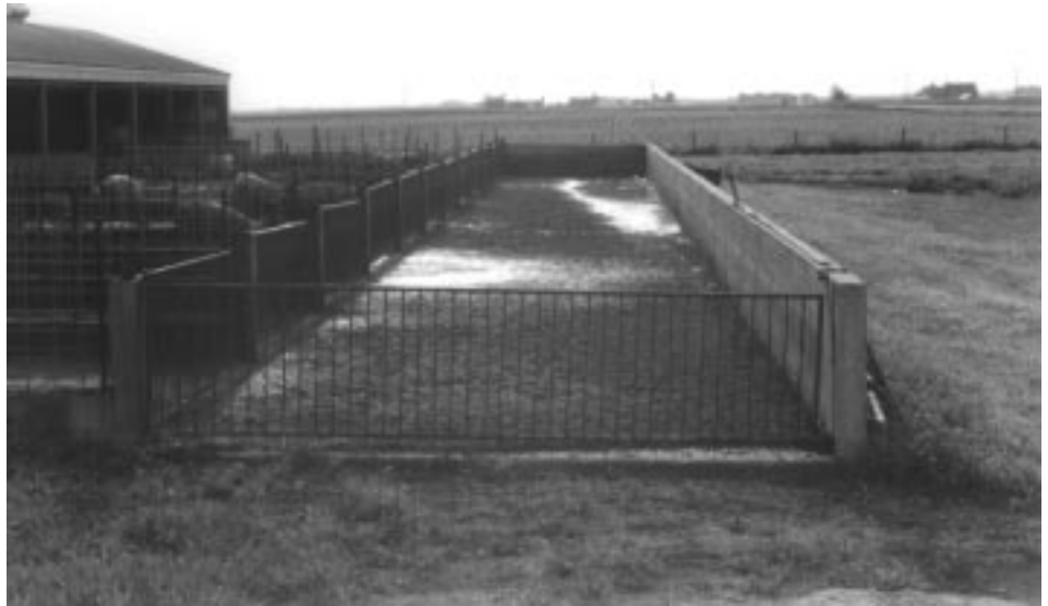
The settling area is 33 percent of the lot drainage area. Notice the lip from the lots to the alley. The alley needs frequent cleaning.
