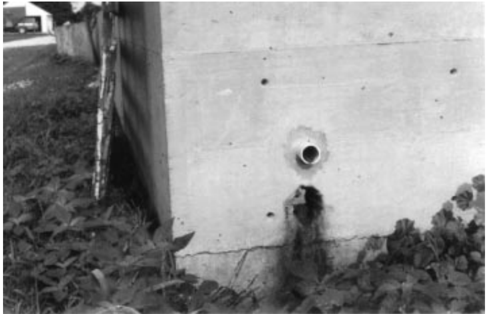
A hole at floor level in the end of the alley is the outlet for liquids.
