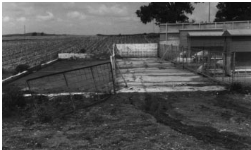
The apron next to, and just above the collection alley is used for vehicle access to fill feeders. Solids can be temporarily pushed against the concrete wall at the far end.
