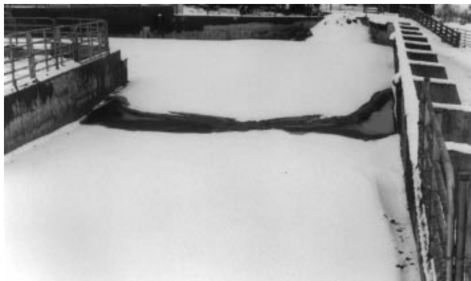
One leg of the comma-shaped pit is an access ramp allowing machinery to enter the pit.
