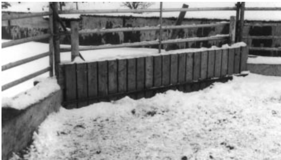
Vertical 2-by-4's make a porous dam in a lot corner to retain solids. Liquids bypass the pit via an intake behind the dam, and a short drain line.
