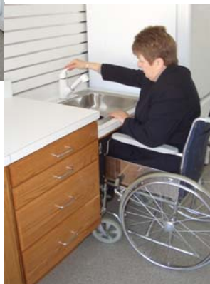
Step 4: Replace the deep sink with a shallow one, so faucets are easy to reach.
