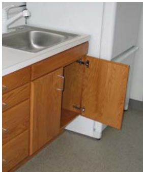
Step 1: Remove doors from standard cabinet.
