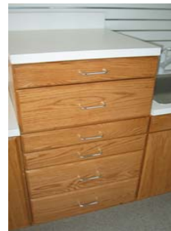
Top boxes of various sizes can be added to change counter heights.
