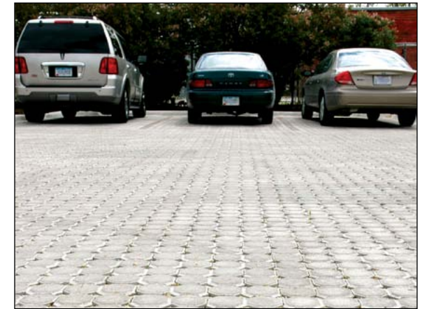
Permeable pavers allow water to seep through instead of running off into storm sewers.
