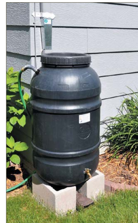
Rain barrels collect rainwater from eaves and holds it for lawn or garden watering when needed.
